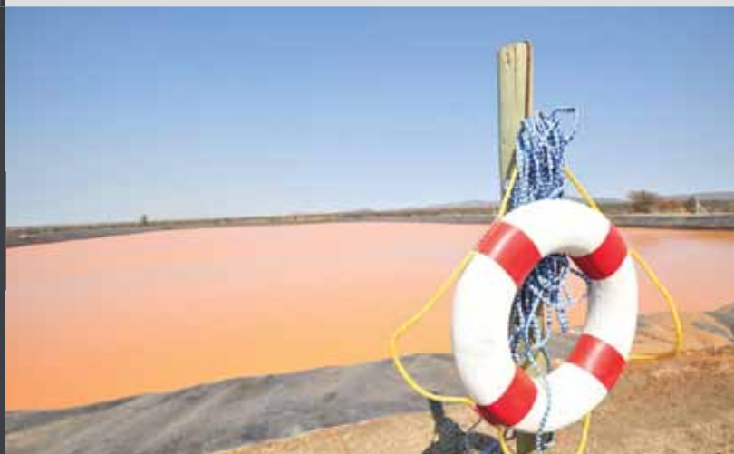
Pollution control dam
