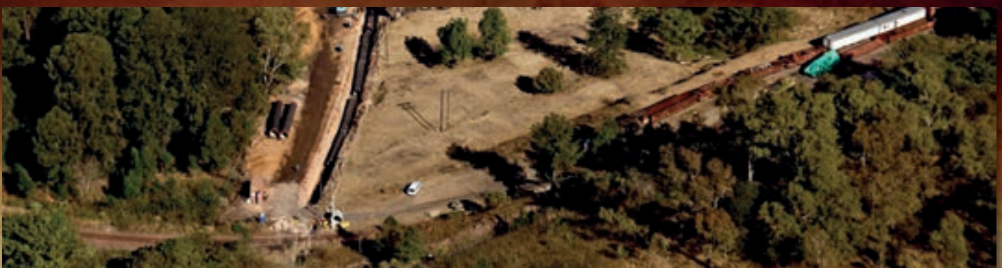
Aqueduct water pipe replacement project.
