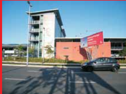
KING SHAKA INTERNATIONAL AIRPORT OFFICE BUILDING AND PARKADE
