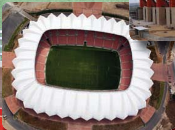
Nelson Mandela Bay Stadium, Port Elizabeth
