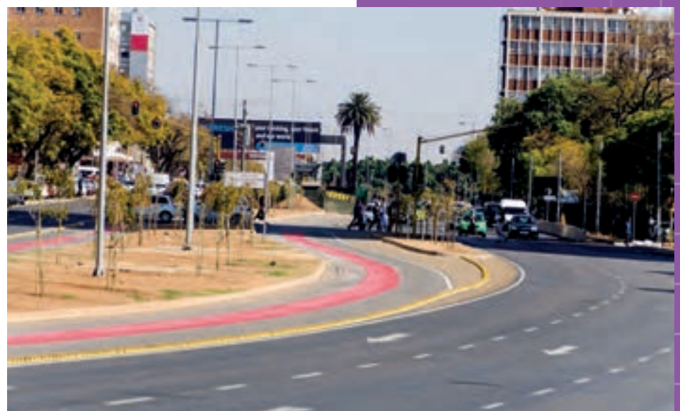
Completed busway on Nana Sita Street in the Pretoria CBD.
