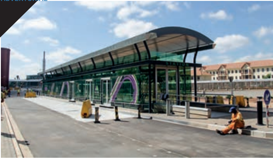
A completed A Re Yeng station in Hatfield.
