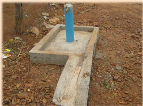
One of the water taps of the reticulation water project in Muyexe that has been completed recently to improve water supply to the community.
